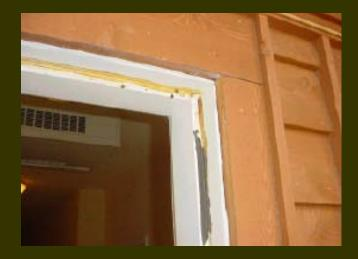
Exterior Door Missing Weather Stripping
