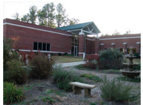
South Piedmont Community College implemented a $376,481 energy saving performance contract in August 2004.
