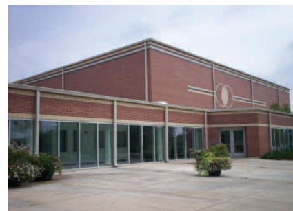
Columbus County Schools launched a guaranteed energy saving contract in June 2003. The project included energy efficiency upgrades with a total project cost of $1,990,000.
