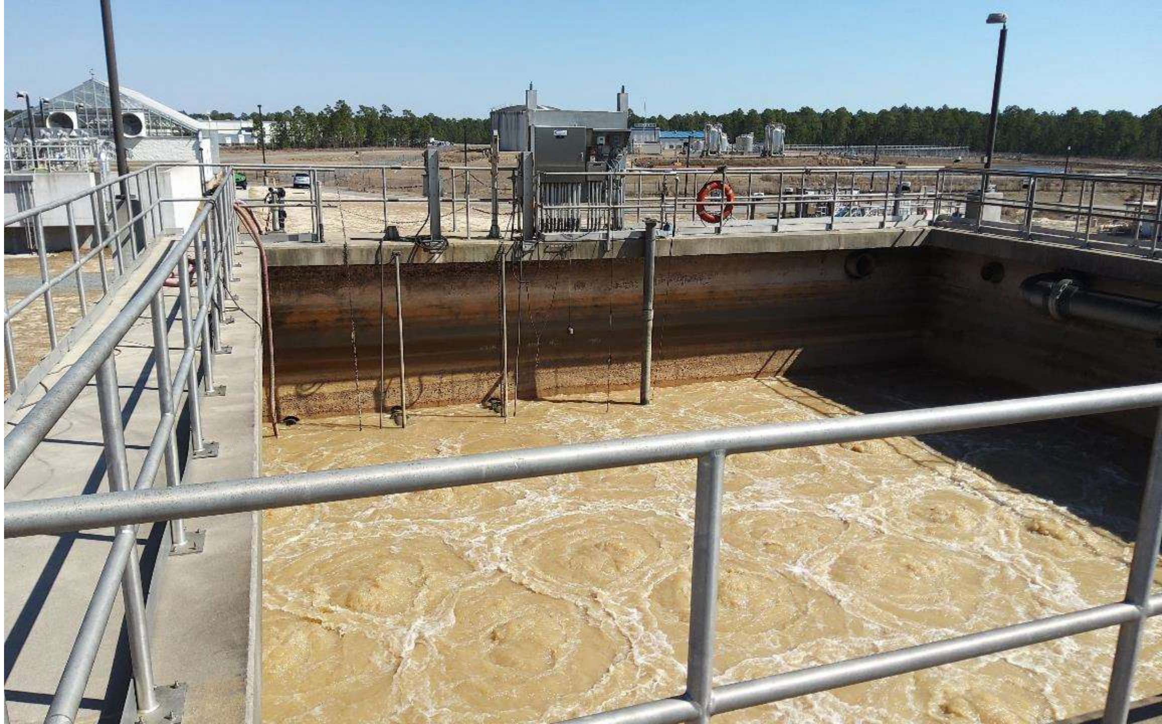
A View of the EQ basin from the screen and grit station (off camera behind).
